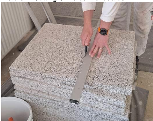
Picture 1: Cutting Clima control boards
